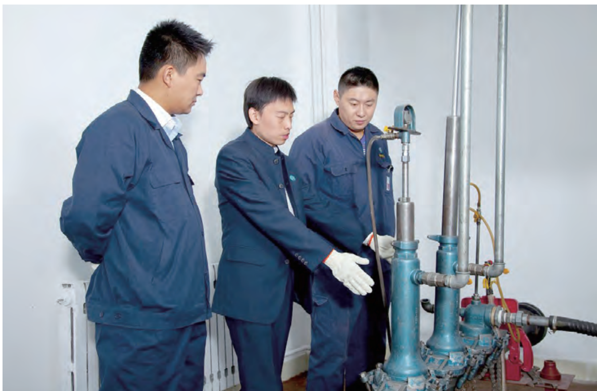
燃氣管網技術培訓 Technical Training on Gas Network
