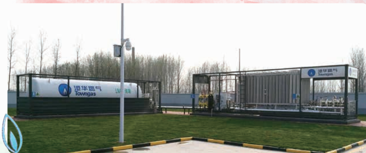
This innovative skid-mounted small liquefied natural gas transition station was developed and designed by our Engineering Department. We have obtained a national invention patent and three utility model patents for the design.
